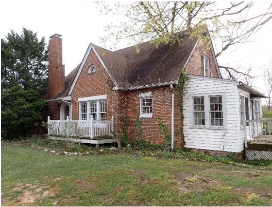
Picture 1 Front of subject house
