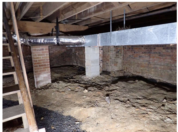
Picture 18 Right half basement/cellar, dirt floor, functional drain system
