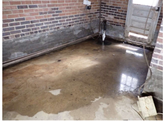
Picture 20 Standing water at basement, left half
